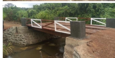
Second picture: Side view of the ARILE bridge after construction work.
